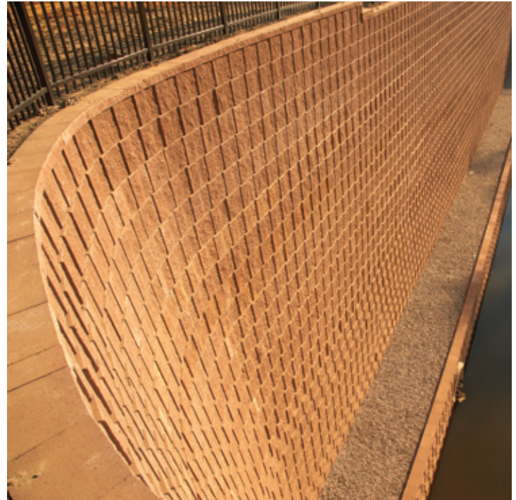
The aesthetics of the Landmark retaining wall system and the nearly vertical system batter were both needed by the designers of this retention pond near a high-profile shopping area.
