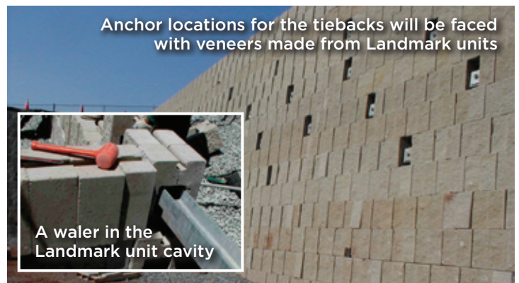
Installation of the tiebacks
